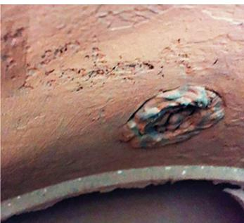
Chaplets are usually comprised of different metallurgy from the metal being poured and can create a weak area if left in place. Image 2 shows areas that were either utilized for chaplets or are core sand clean-out plugs, which were excavated and welded.
