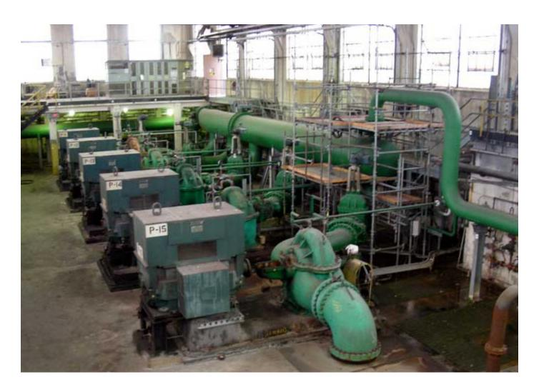
Positioned on the shores of Lake Michigan are two stations that contain cooling water pumps which feed cooling water to BP's Whiting Refinery. The #1 water station contains four IR 24 HV pumps, which are large, single-stage, double-suction, horizontal split case pumps. Four pumps in station #1 (P-11, P-12, P-13, and P-14 in the photo below) are unique in that they were designed with a bottom-suction configuration.
