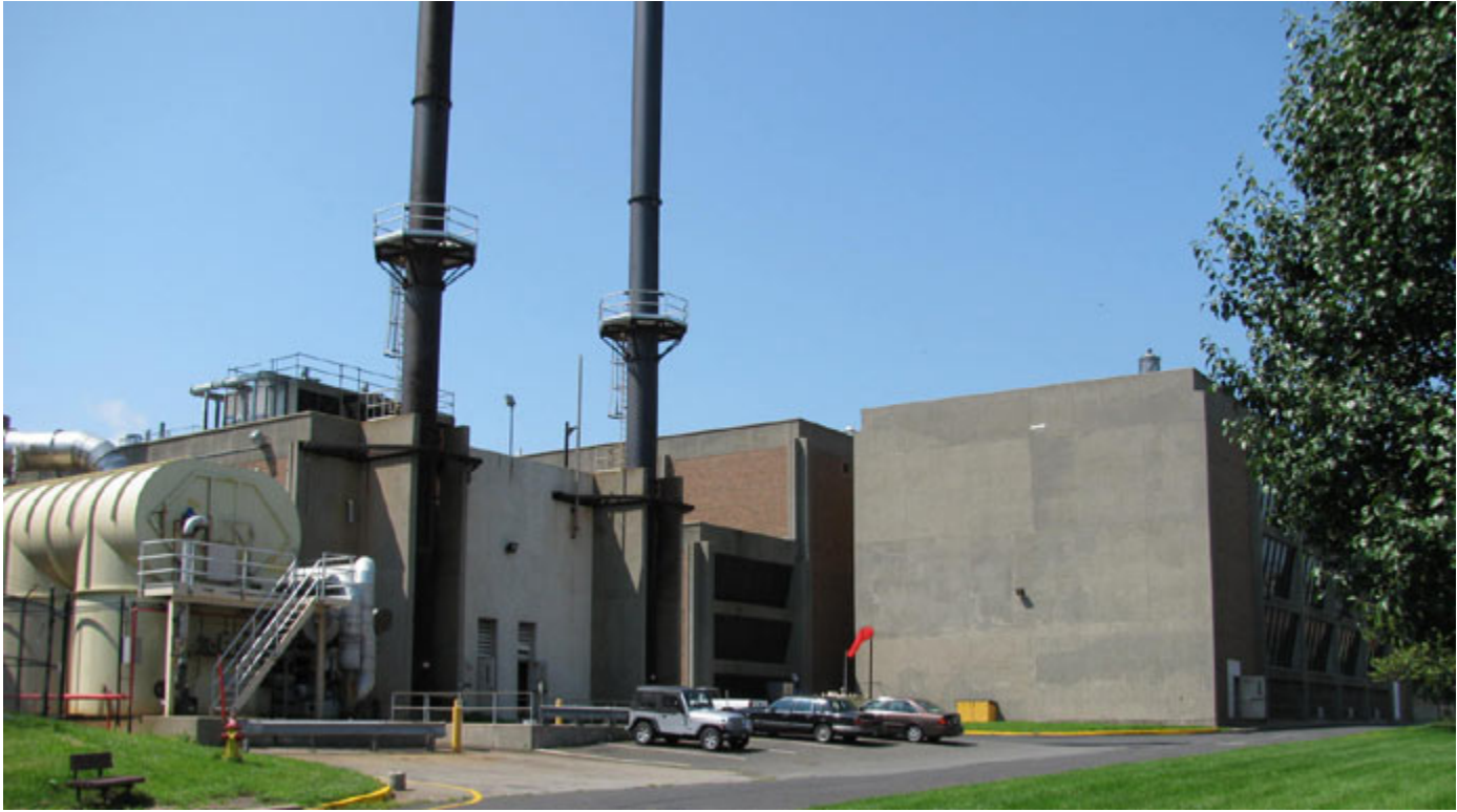
Facility's boiler house
