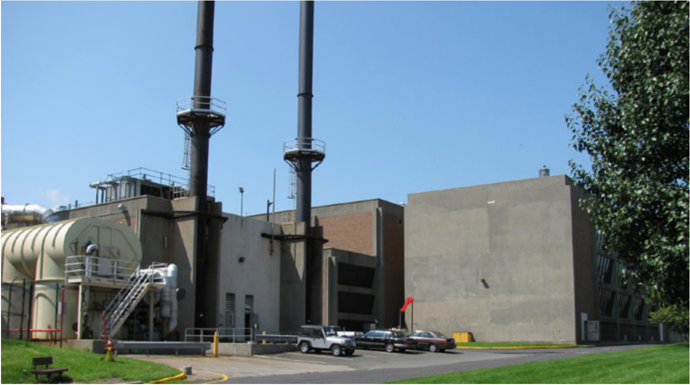
Facility's boiler house
