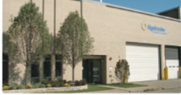
HydroAire, Inc. (40th Street Shop) | Chicago, Illinois
