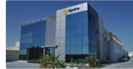
Hydro Middle East, Inc. | Dubai, United Arab Emirates
