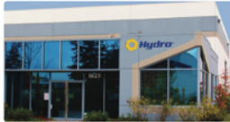
Hydro Richards, Inc. | British Columbia, Canada
